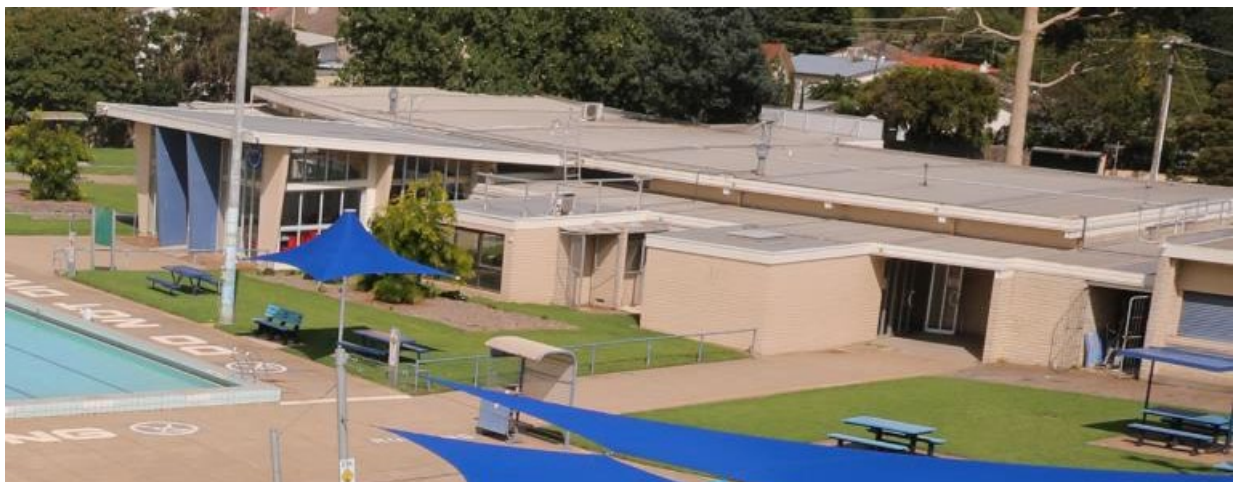
Figure 27. Doveton Pool main building viewed from the top of the water slide to the west. Note clerestory windows which appear to have been covered up above the former covered (now enclosed) walkway and additions to the rear of the building beyond the line of the original concrete block piers. (Source: Tract Consultants 2020)
