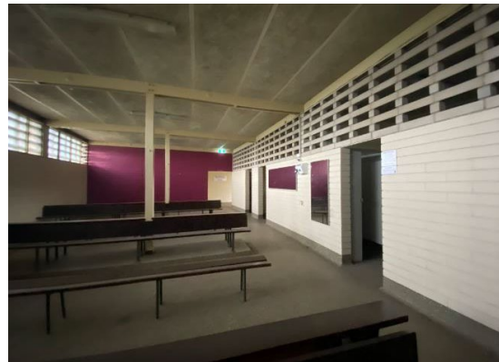
Figure 31. Female changerooms showing bench seating. Showers are located behind the part-height concrete brick wall to the right of image. Note more continuous areas of openwork header and stretcher concrete blocks to upper section of wall. (Source: Context, 2020)
