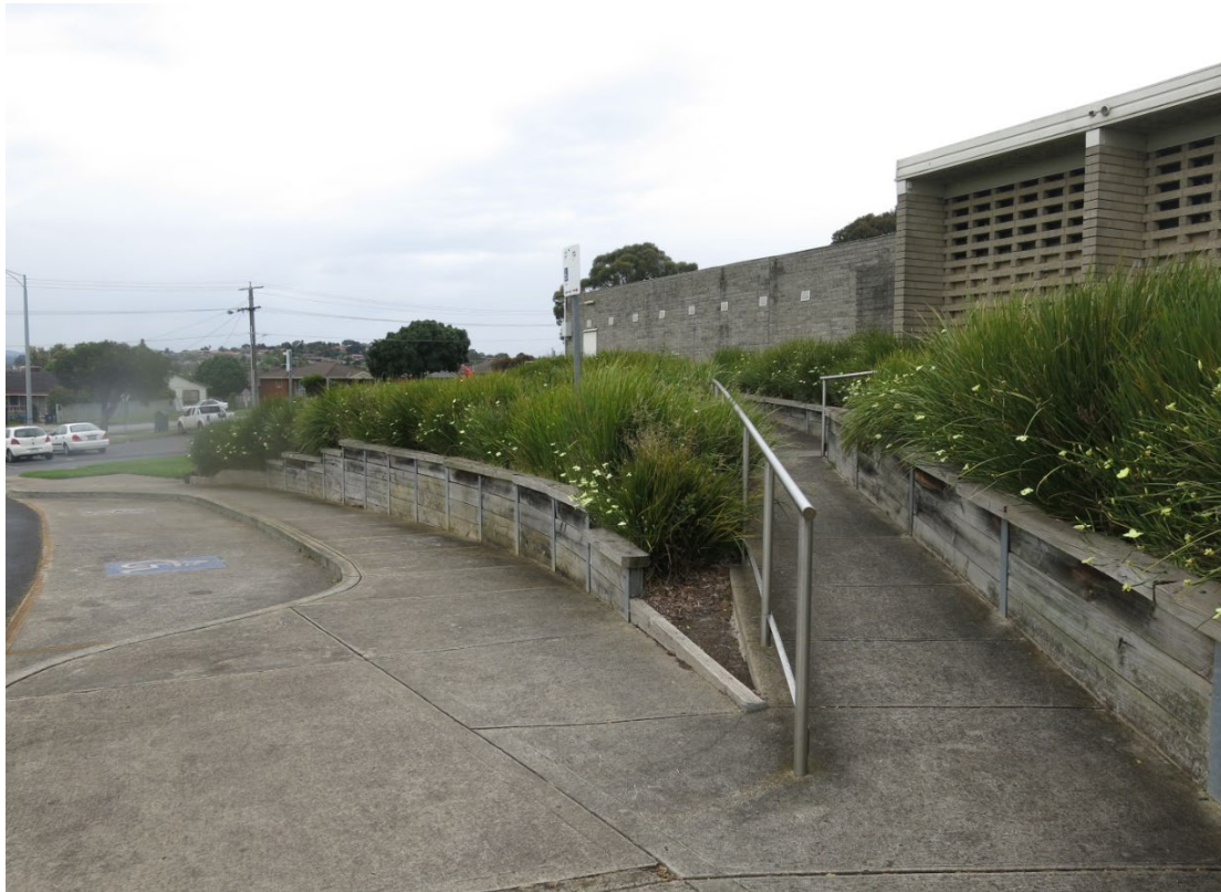
Figure 25. Detail of ramp and garden beds with timber retaining walls in front of 1977 addition and northern end of facilities building. (Source: Context)
