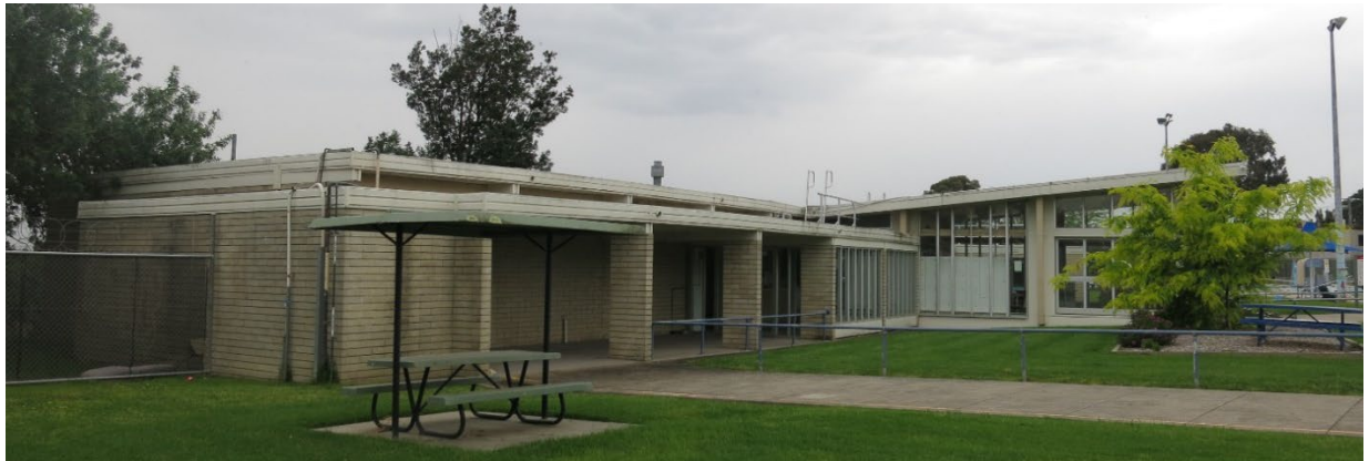
Figure 26. Doveton Pool main building viewed from the southwest. Note smooth-faced concrete block piers and recessed split faced concrete block wall (left) and glazed corridor and projecting skillion-roofed extension to centre of building (right) built in 1993. (Source: Context 2020)
